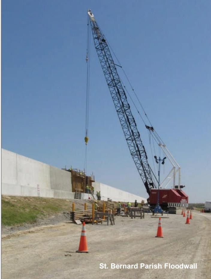
The last monolith is placed into the St. Bernard floodwall, a perimeter wall that runs 23 miles through the parish. The floodwall is anchored beneath by more than 42,000 H-piles driven to depths of -40 feet to -166 feet to provide stability and strength to the floodwall.
