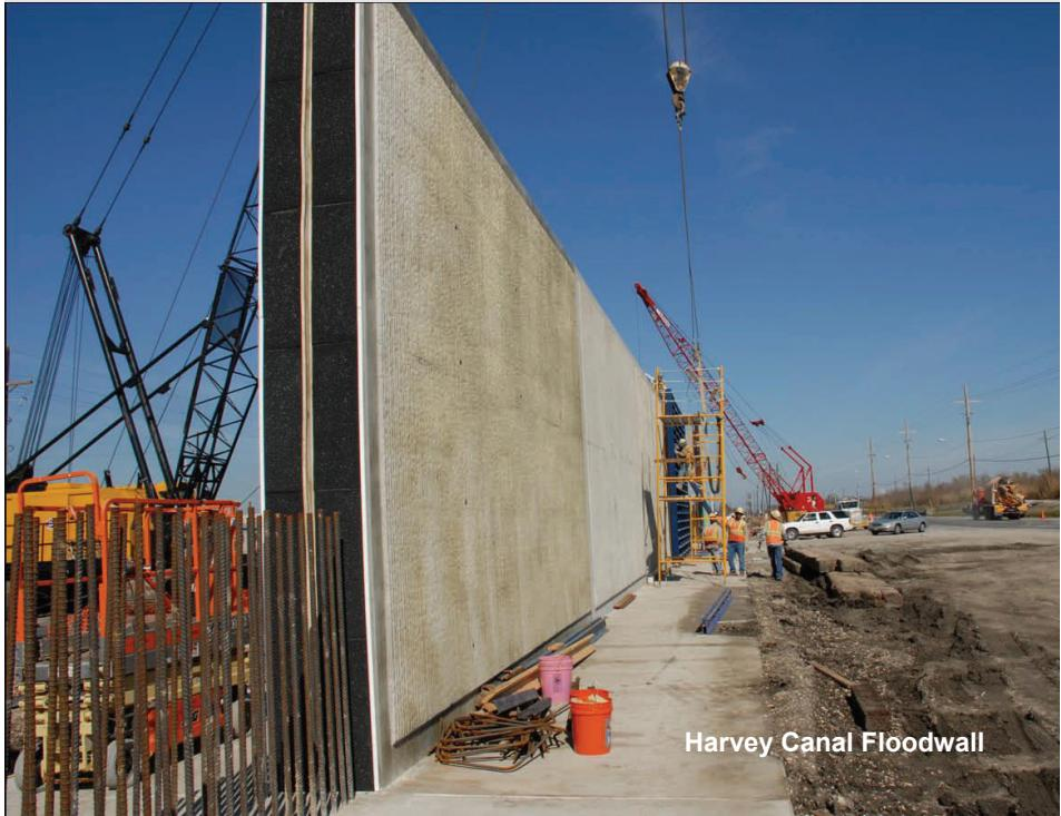
The Harvey Canal floodwall (now complete) on the West Bank stands 15-19 feet tall with steel pilings as deep as a 12-story building.
