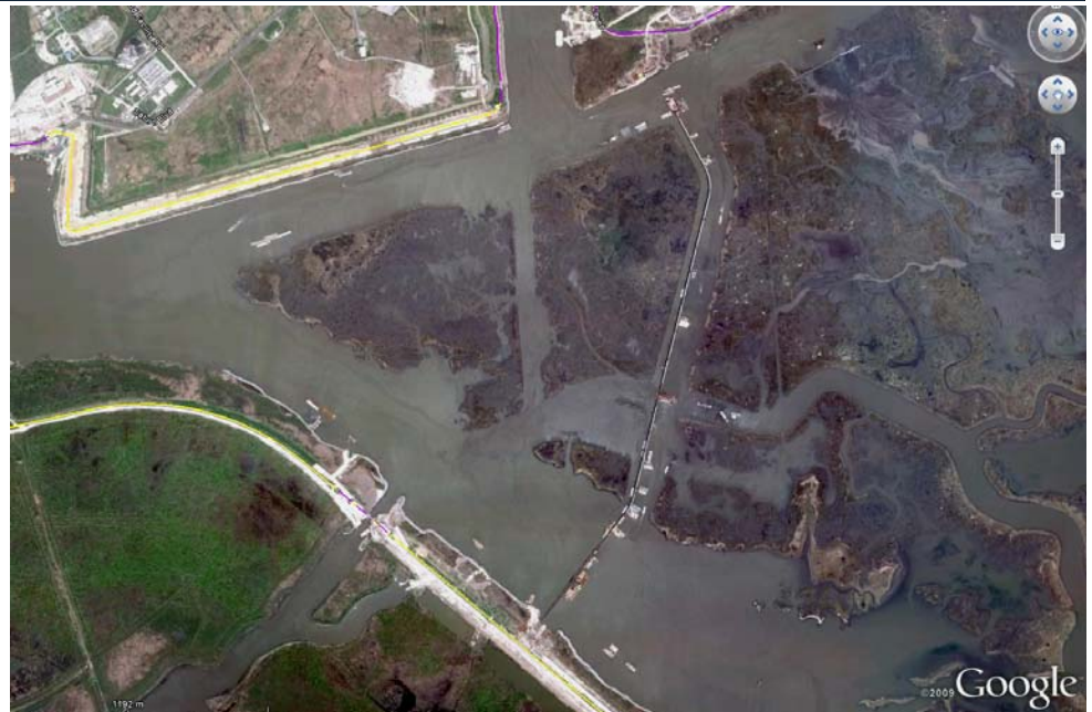
This image from Google Earth shows the IHNC Surge Barrier spanning nearly two miles - from the Gulf Intracoastal Waterway (at Michoud) to across the MRGO. When completed, the project will include gates at the GIWW and at Bayou Bienvenue. 100-year level risk reduction features are expected for June 2011.
