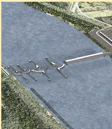
Artist's conception of the massive West Closure Complex surge barrier gates and pump station crossing the Gulf Intracoastal Waterway.
