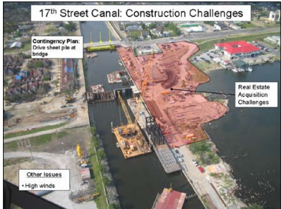
This graphic of the 17th Street Canal project shows challenges facing pump installation. The U.S. Army Corps of Engineers had to acquire the pink-shaded area before construction could begin. Other delays were due to high winds on the construction site, and the need to purchase or lease other properties. (USACE photo)
