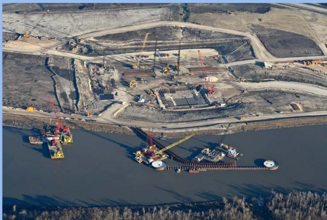
West Closure Complex - Under Construction
