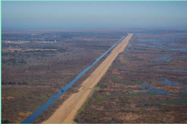
Levee raise - St. Bernard Parish - Complete
