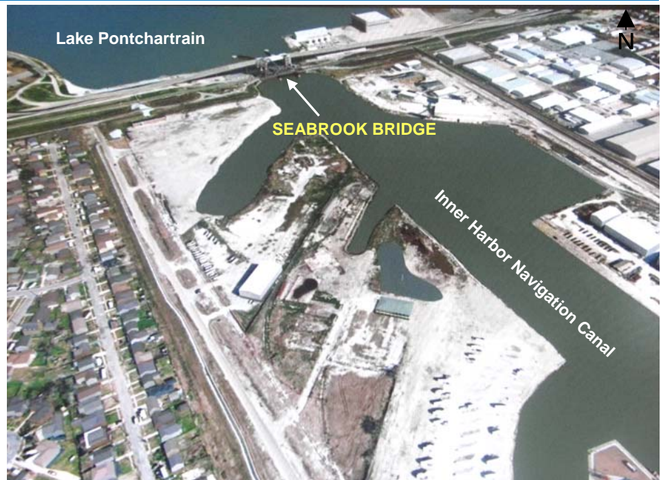
This aerial view of the IHNC at the Seabrook Bridge was taken from the Corps' website animation that illustrates the three Seabrook Floodgate alternatives. To view the animation, go to: http://www.mvn.usace.army.mil/pao/videos/pao_videos.asp
