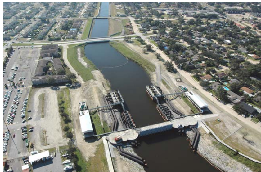
London Ave. temporary pump station
