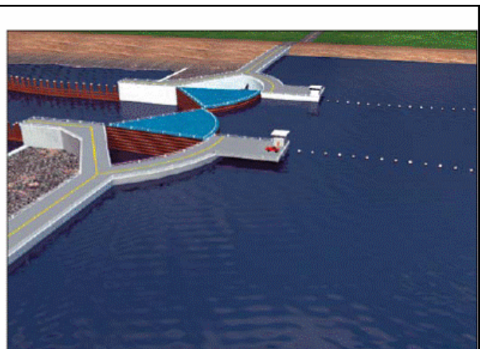
GIWW Structure Closed for Flood Control
