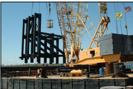
Closure gates under construction at 17th Street Canal. (USACE Photo)
