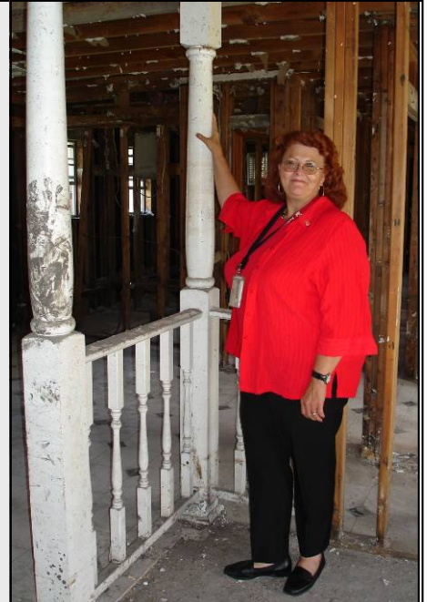
Sherry Scott inspects her gutted home in Chalmette recently. She had just moved into her home when Katrina flooded it. (USACE Photo by Susan Solomon)
