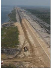
Millions of cubic yards of soil will be needed to restore and build the levee system in the greater New Orleans area; and all soil used is stringently tested. (USACE Photo)
