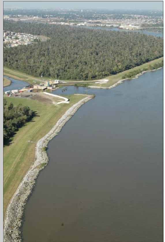
New Estelle Pump Station and levee
