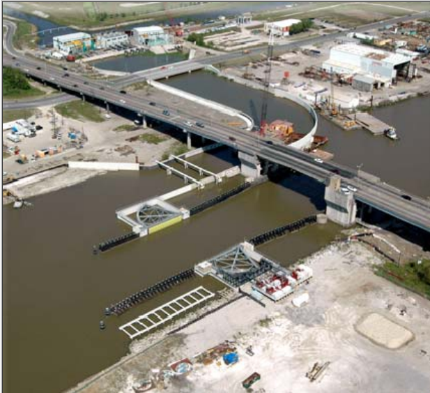
Harvey Canal Sector Gate Complex Station
