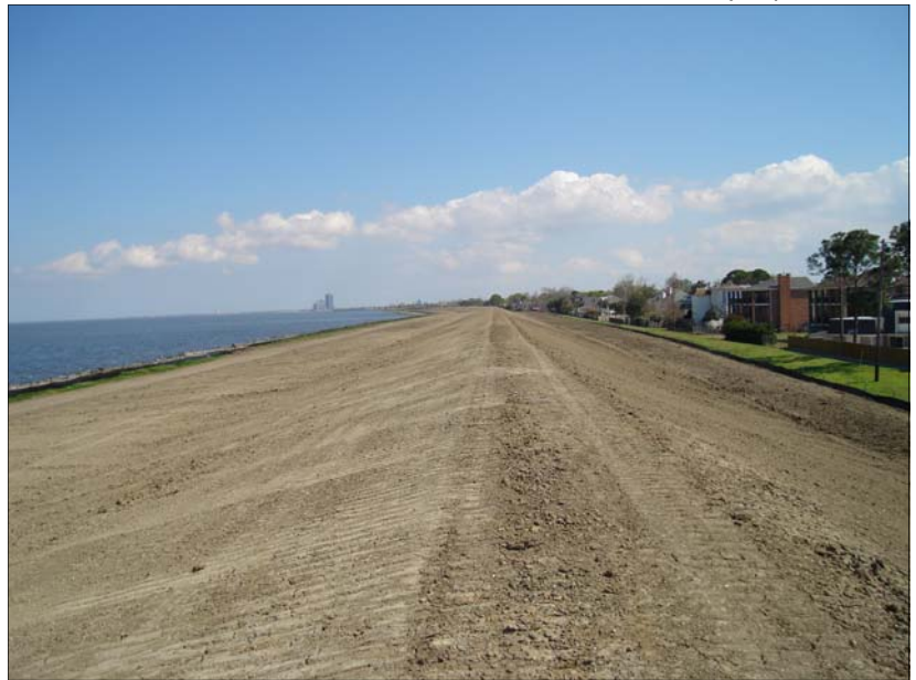
This levee has been “fine dressed” and awaits the turfing process.
