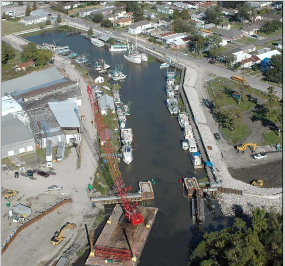
Company Canal floodgates under construction
