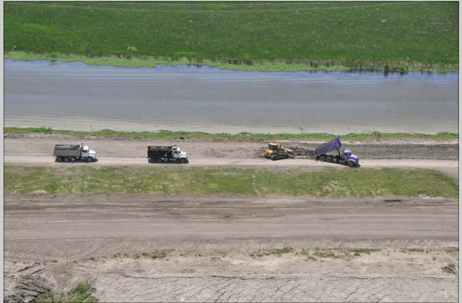
Trucks deliver clay for the levee at Lake Cataouatche
