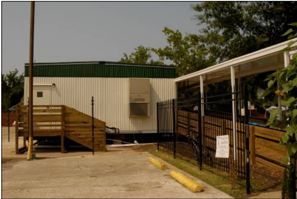
Back view of Ecole Bilingue in New Orleans. (USACE photo)
