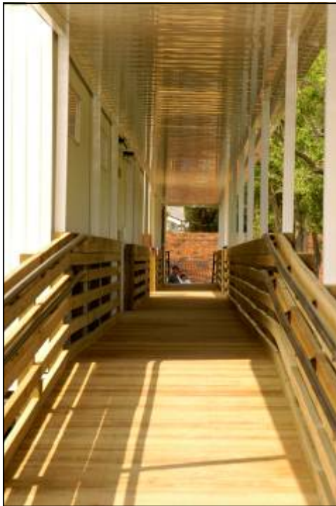
Ramp walkway (top) and classroom (right) at Ecole Bilingue in New Orleans. (USACE photos)
