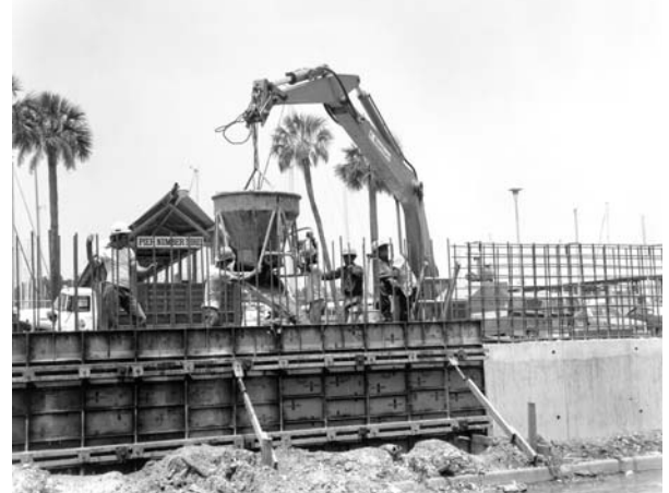
Feb. 1979 Construction of the New Orleans Marina flowwall.
