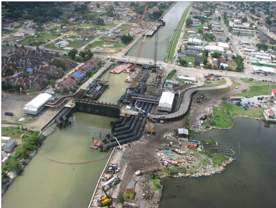
17th Street Canal — July 2007
