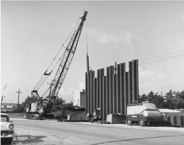
Aug. 1967 Applying sheet piling at France Road at IHNC.
