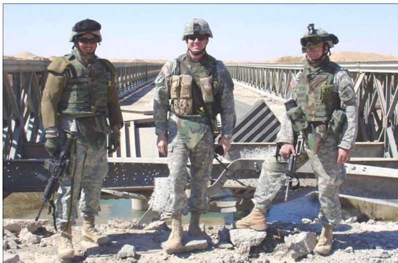
Maj. Nazarko, center, poses with his team mates in front of a bridge damaged by insurgents in Falluja, Iraq. At left is Specialist Donald Heiney, and at right Specialist Joshua Coster. "We were there to assess the bridge for repairs," said Nazarko. (USACE Photo)
