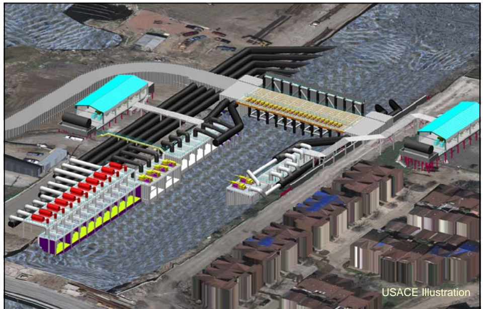
This is an artist's rendering depicting what the 17th Street Canal closure gates and pumps will look like after the 11 new pumps (in red) are installed. The pumps will have the capacity to pump 7,600 cfs of water from the canal into Lake Pontchartrain when the gates are closed because of storm surge.
