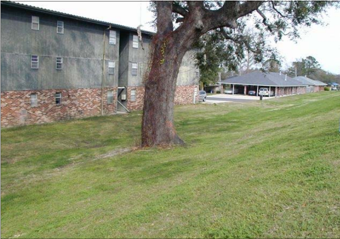
Trees growing in the levee “toe” undermine the integrity of a levee and leave it vulnerable in a storm event or hurricane.
