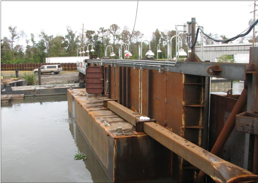
The Company Canal “barge gate” acts as an interim measure to reduce surge into the canal during storms. (USACE Photo)
