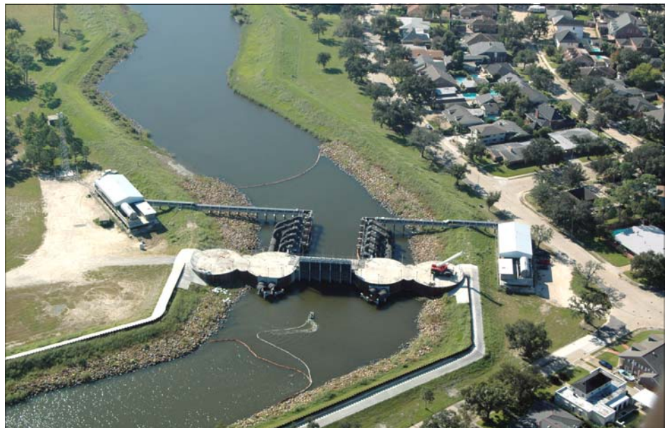
Interim pumps and gates at the Orleans Ave. Outfall Canal (above) were authorized and funded through the 4th Emergency Supplemental Appropriations Act, as were the pumps and gates at the 17th Street and London Ave. Canals. This type of funding is outside the normal Corps budgetary process. (USACE Photo)
