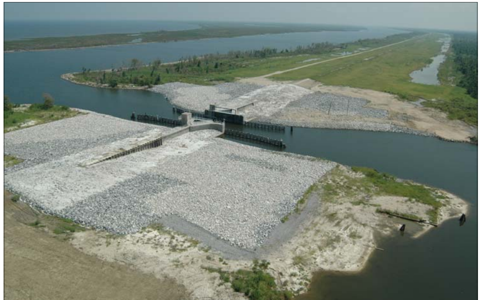
Bayou Dupre floodgate at the Mississippi River Gulf Outlet, above, was heavily armored following Hurricane Katrina. (USACE Photo)
