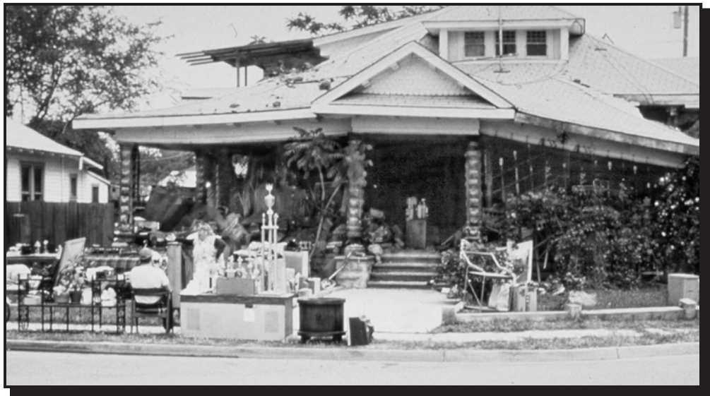
Damage from magnitude 6.7 earthquake
