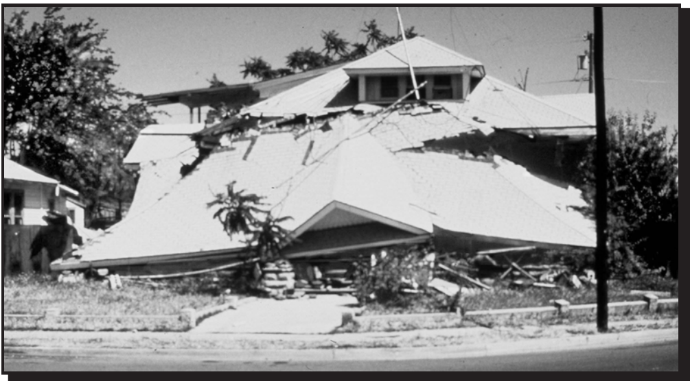
Additional damage from aftershocks
