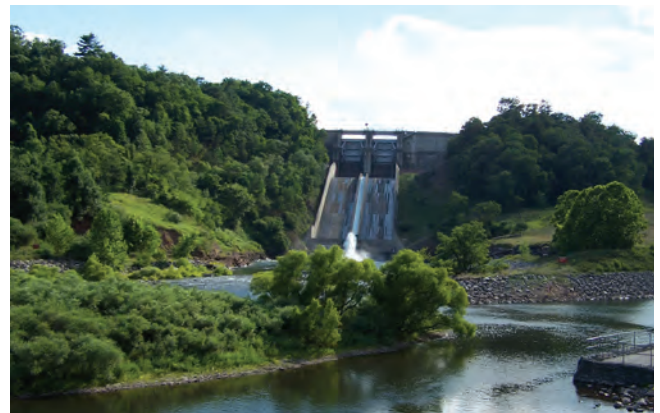
Pennsylvania spillway. Photo courtesy of Frank Borsuk.
