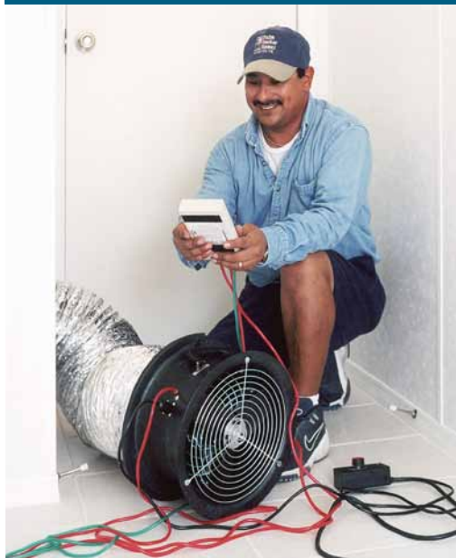
Your contractor will test the leakiness of the ducts with a duct blaster test (Source: NREL).
