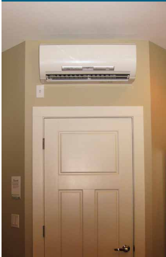
Ductless heat pumps can provide efficient zoned heating and cooling.
