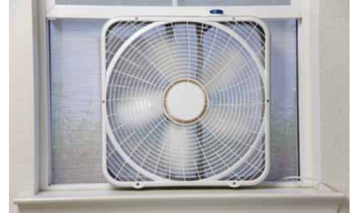
Window fans pull hot air out of the home.
