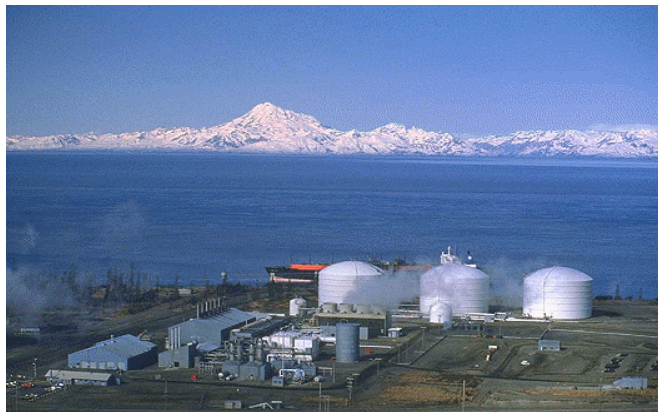
Figure 5. LNG Liquefaction Facility in Kenai, Alaska
