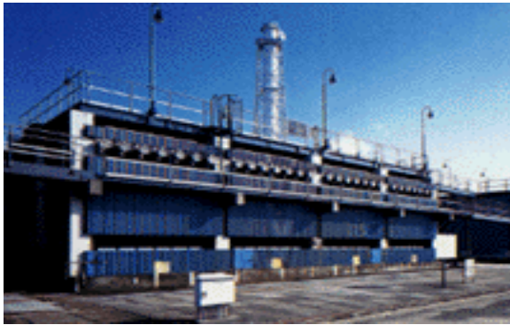
Figure 25. Open Rack Vaporizer
