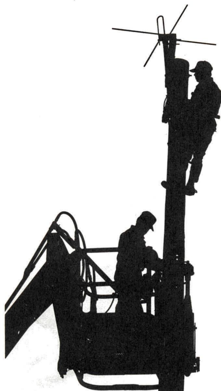
High over the flight ramp, SSgt. Dennis Cierpial, 905th CF (top) and SSgt. George Nalesnik, 901st CF, replace an old SAC VHF radio antenna with a new UHF antenna.
