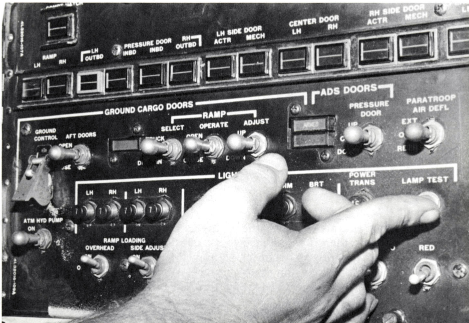
CONTROL PANEL — Part of the controls that operate the hydraulic system for the rear doors and ramp.
