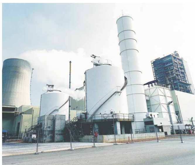
ELCOGAS IGCC Plant is a 350MW power plant located in Puertollano, Spain. Coal gasification and extensive gas cleaning prior to combustion means that atmospheric pollutant emissions at IGCC plant are as low as those of natural gas combined cycle plant.
