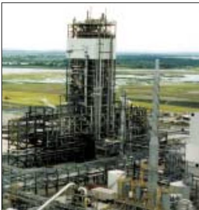
Tampa Electric Company's 250-MWe Polk Power Station, Unit 1 IGCC facility
