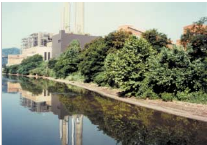
American Electric Power's 600-MWe Cardinal Plant in Brilliant, Ohio
