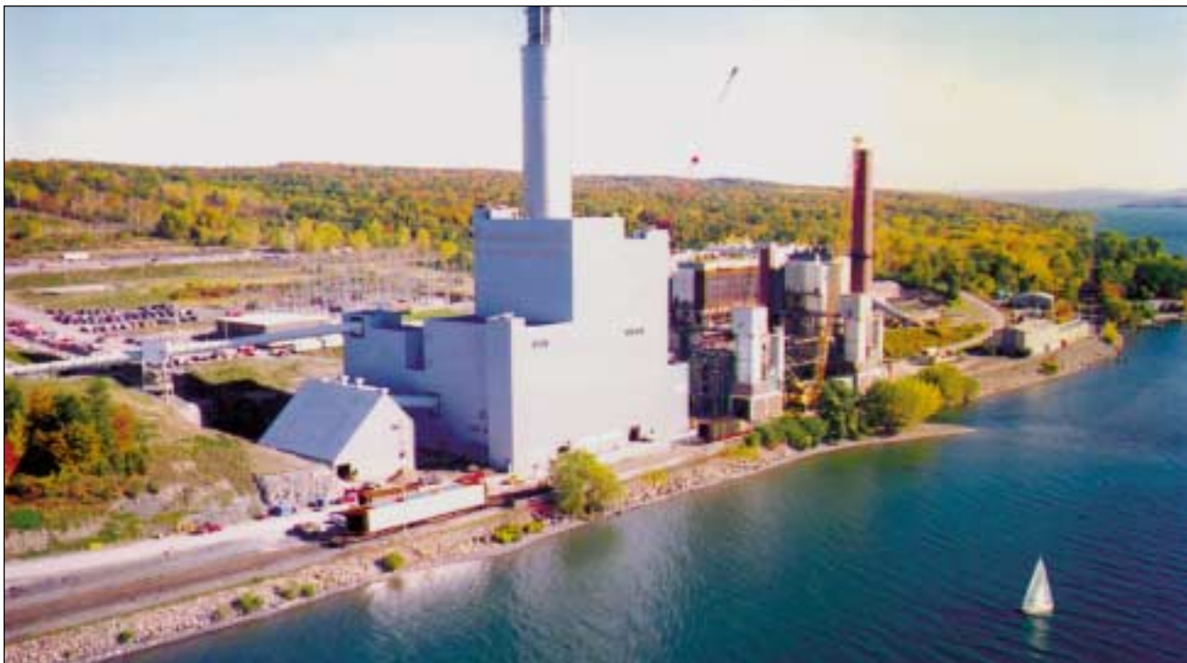
New York State Electric & Gas Corporation's Milliken Station hosted a Clean Coal Technology Project to demonstrate high efficiency SO 2 , NO x , and particulate control without discharge of solid or liquid wastes
