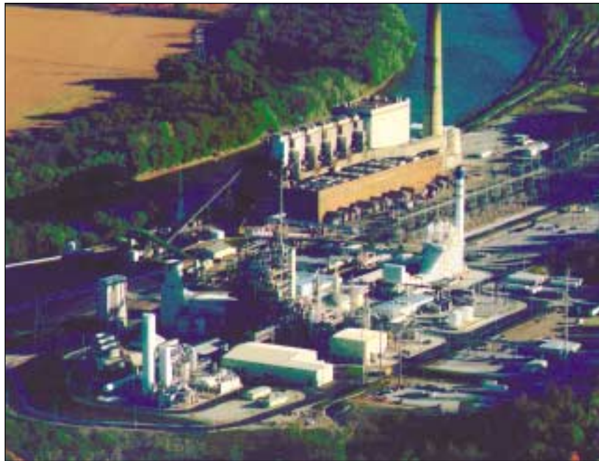
Wabash River Generating Station was repowered with a 262-MWe IGCC unit shown here
