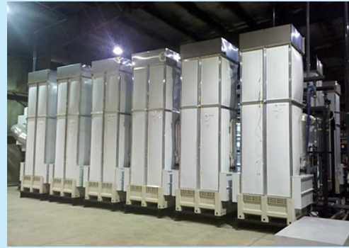
An AltelaRain® desalination unit and water treatment towers.
