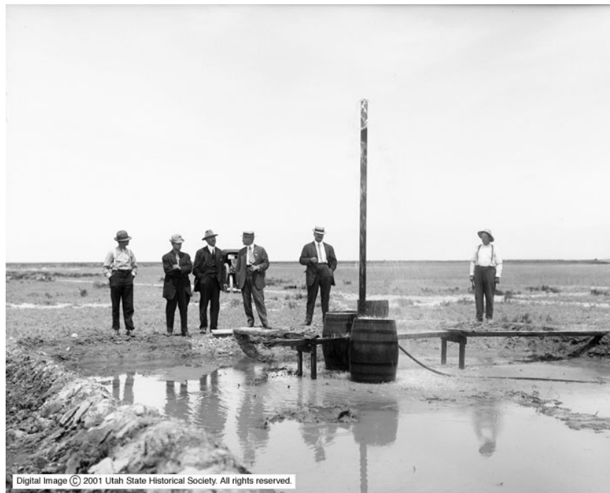
Figure 3 - Highland Improvement Company Well (1914)
