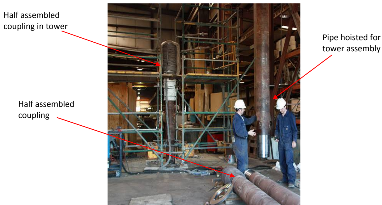
Figure 4.5 – Preparation for Second Shrink-Fit in Assembly Tower
