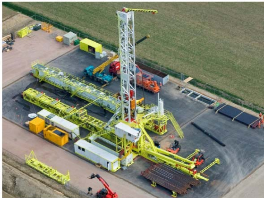
Figure 1, LOC 400 Drilling on location in the Netherlands 2010
