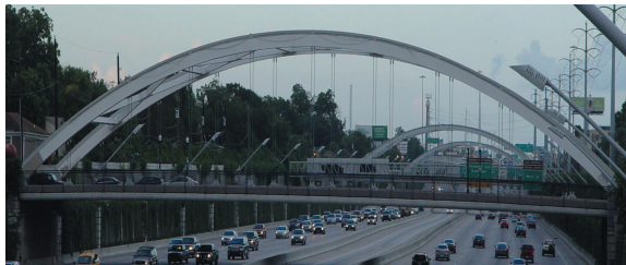
(a) Arch Bridge across US 59 and Mandell St
