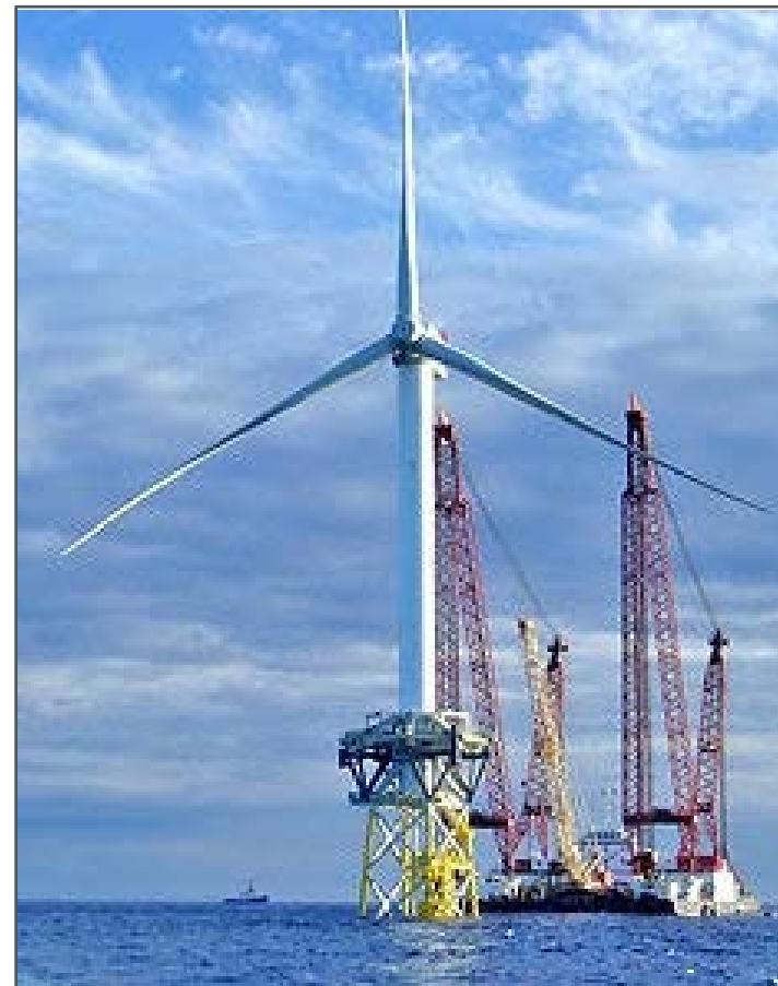
Repower 5MW Demonstration at Beatrice Four-pile jacket
