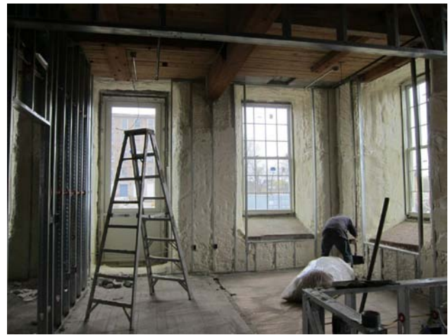
Figure 21. Tapered window opening jamb detail and interior view (sill left uninsulated)
