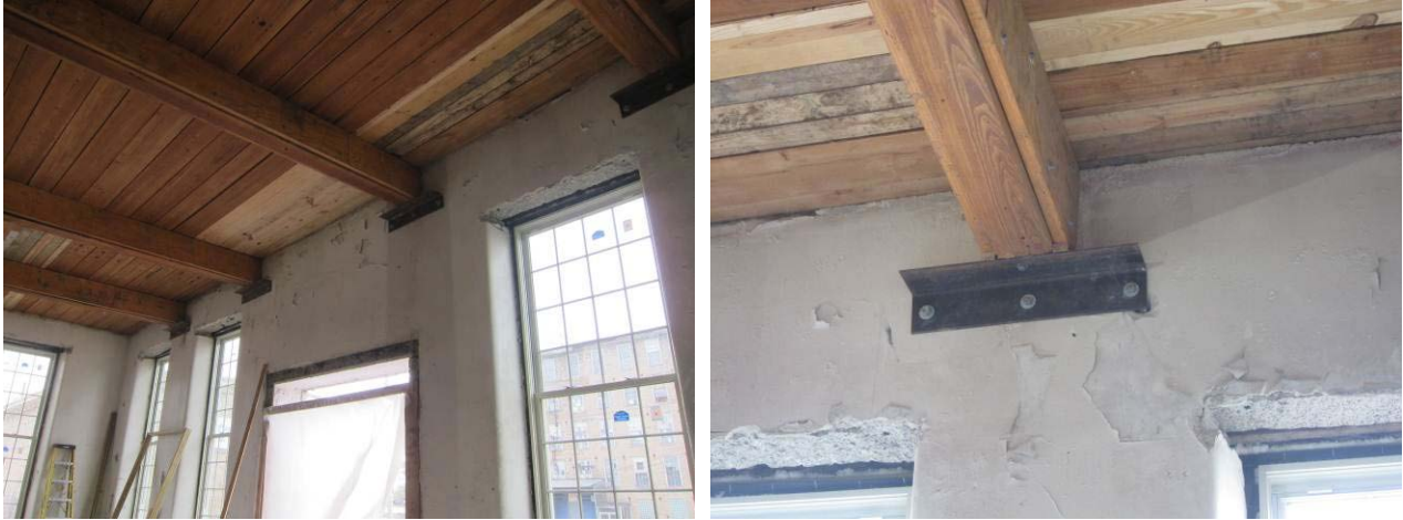
Figure 16. Steel angle bolted to masonry to transfer load out of beam pocket
