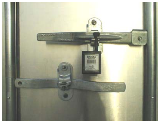
Figure A.2.8. Detail of Simulated Container Door, Handles, and Keeper Bars
