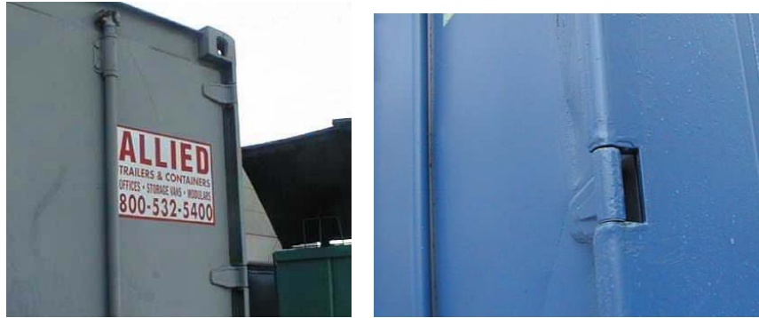
Figure A.5.8. Hinge Region of ISO Cargo Containers
