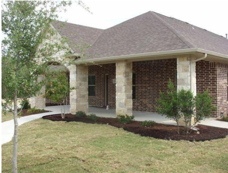
Phase V of Mayberry Gardens, located in Garland, Texas was completed in April 2012.
