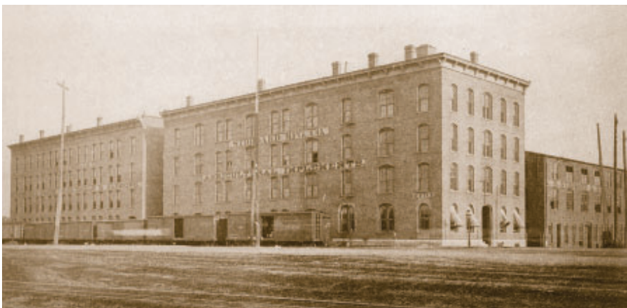
The Stoddard Manufacturing Company on Third and Bainbridge streets built farm machinery until 1905, when it turned to the production of automobiles. At that time, the name changed to the Dayton Motor Car Company. (Dayton Metro Library)
