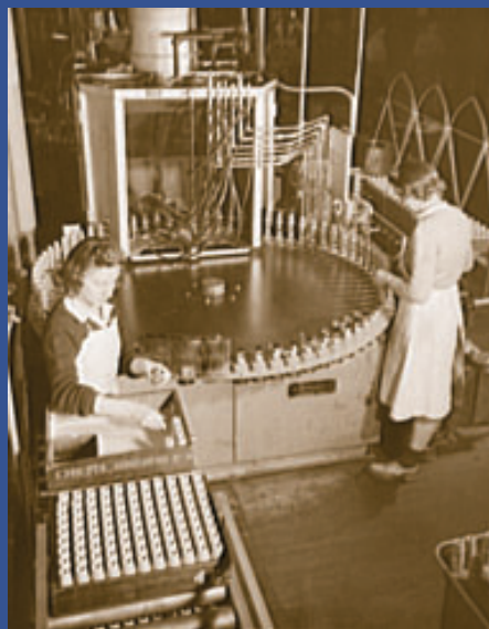
NCR during World War II. A machine paints the exterior and interior of 37-mm high-explosive shells for the war effort. ( Library of Congress, Farm Security Administration, Office of War Information Photograph Collection )
