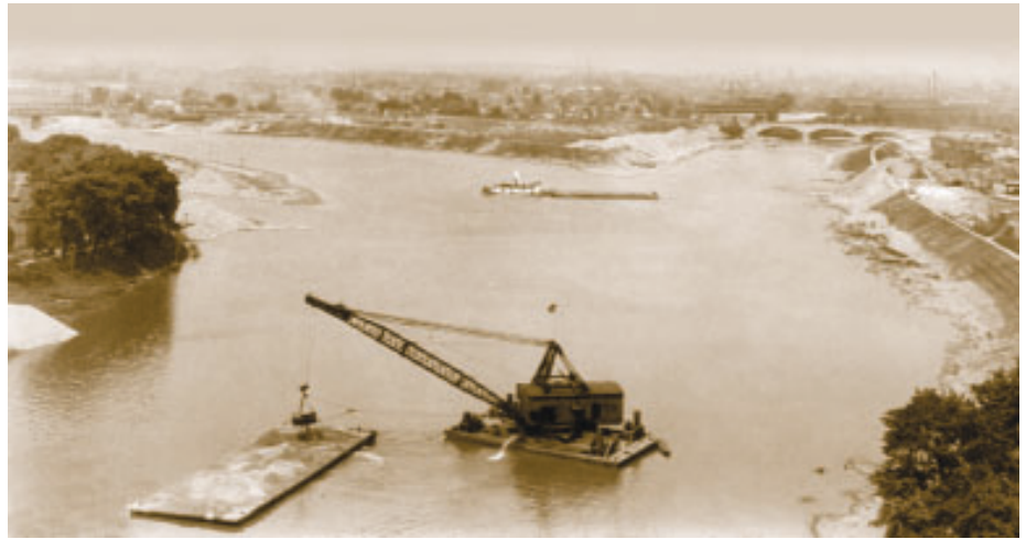
Miami Conservancy District’s steamboat, Dorothy Jean , named for John H. Patterson’s daughter, 1919. The steamboat pushed barges used for dredging the Miami River during construction of the flood control system.
