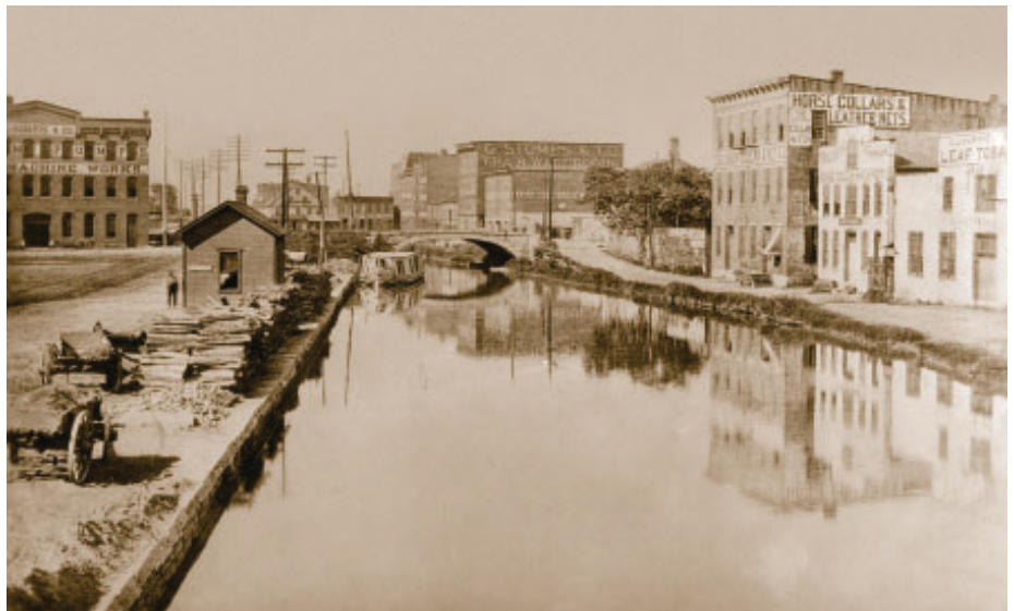
The Miami-Erie Canal reached Dayton in 1829. It was up to 40 feet wide at water level and approximately 4 feet deep. Horses and mules towed heavily laden flat-bottomed boats down the canal. In 1877, the state of Ohio abandoned the canal. Fifty years later, Dayton filled in the bed and replaced it with Patterson Boulevard, named in honor of John H. Patterson, founder of NCR. (Dayton Metro Library)
