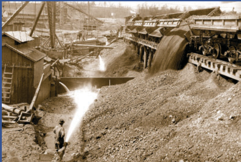
Construction of one of five earthen flood dams in Arthur Morgan's flood control system, 1919. Cost of the construction amounted to more than $30 million.
