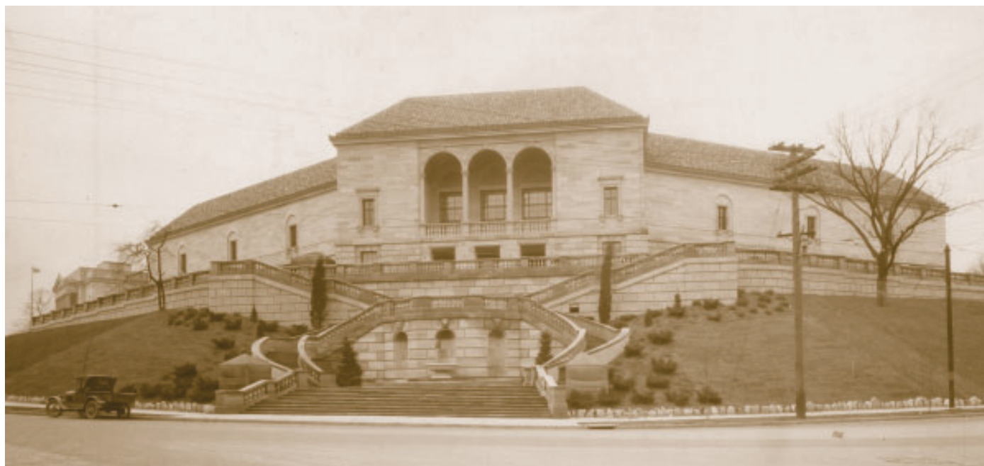
The Dayton Art Institute, founded in 1919 as the Dayton Museum of Fine Arts, was originally located in a downtown mansion. Once its collections outgrew the space, Mrs. Julia Shaw Patterson Carnell funded the construction of a new museum, which was completed in 1930. ( Dayton Metro Library )
