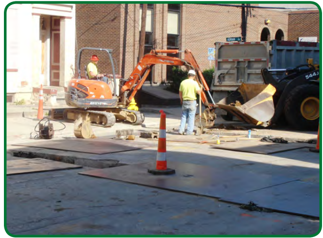
Greater Cincinnati Works does infrastructure work to prepare for the Cincinnati Streetcar. Image courtesy of the city of Cincinnati.
