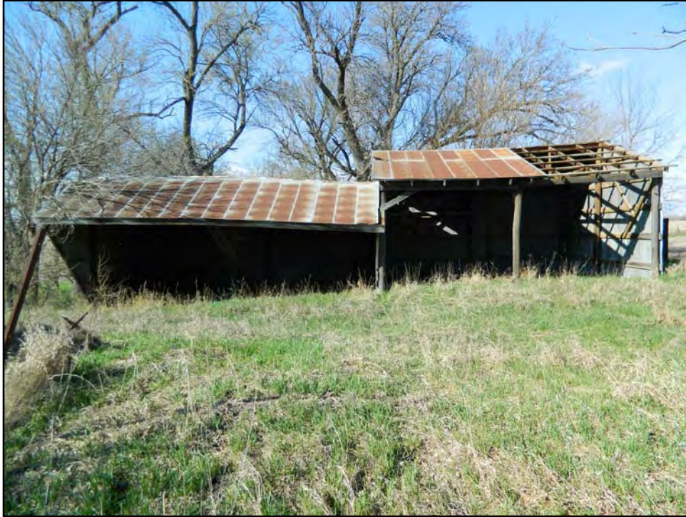
Figure 5.10. Ca. 1955 equipment shed, looking north (RCG&A March 2012).
