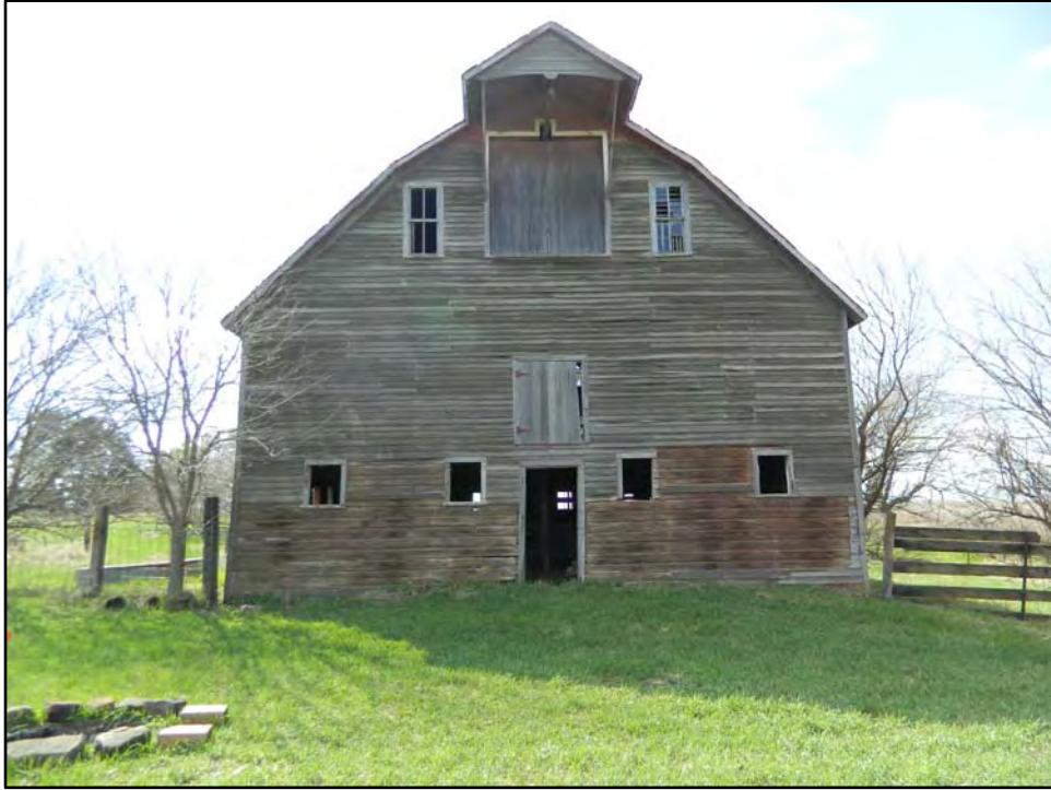
Figure 5.3. East elevation of gambrel roof barn (Feature 1) (RCG&A March 2012).
