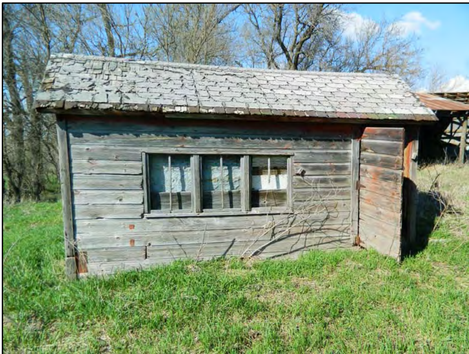
Figure 5.7. South elevation of chicken house (Feature 4) (RCG&A March 2012).
