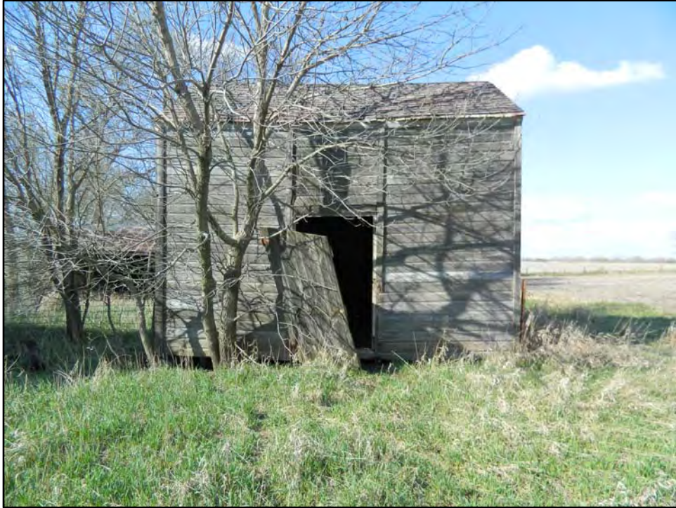
Figure 5.8. South elevation of granary (RCG&A March 2012).
