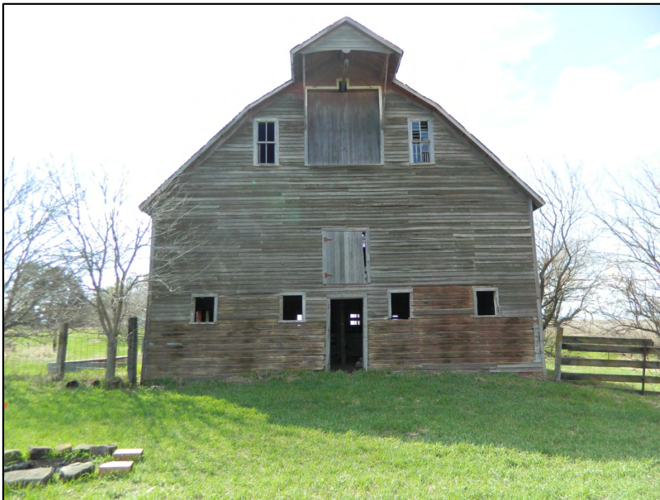
East elevation of gambrel roof barn (Feature 1).
