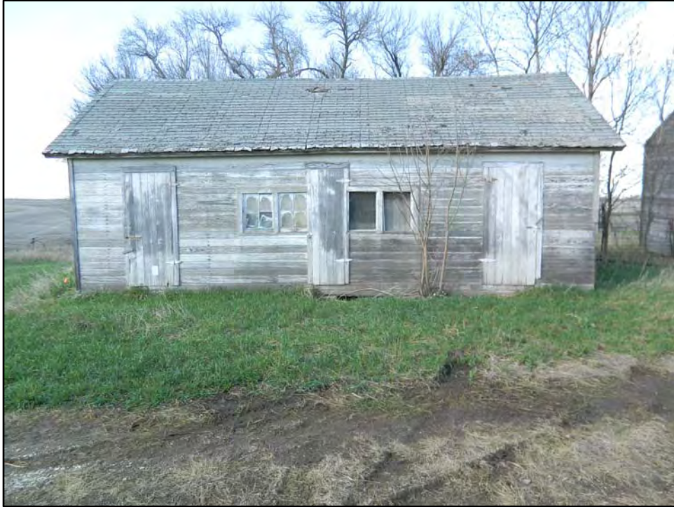
Figure 5.6. South elevation of chicken house (Feature 3) (RCG&A March 2012).
