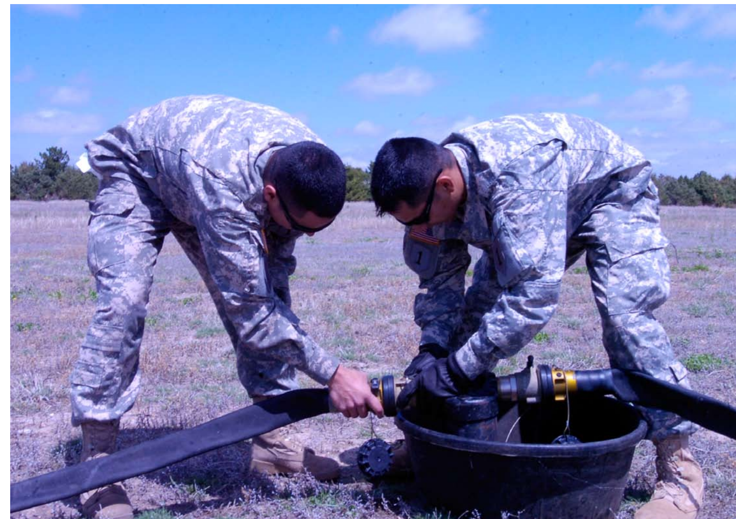
Solid Connection Chief Warrant Officer 3 Jess McGee (left) and Spc. Jaime Reyes connect fuel lines
