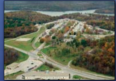
CRANE DIVISION Crane, Indiana
