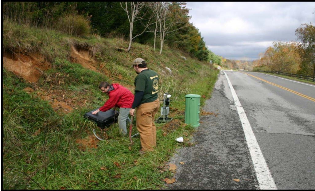
Figure 38 VTTI workers installing radar and camera unit at stop-controlled intersection.
