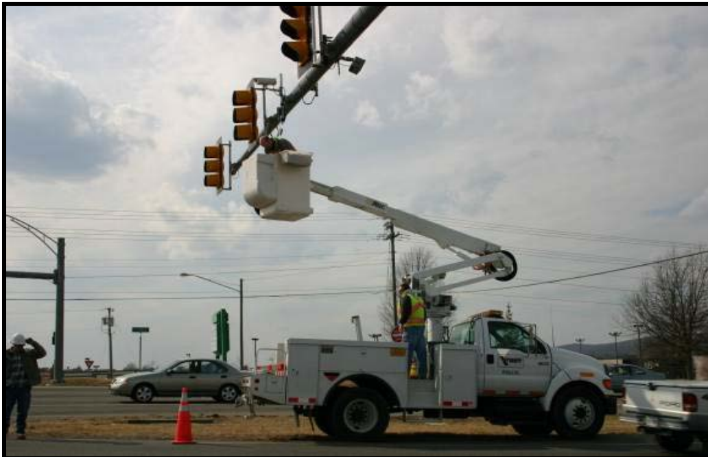
Figure 39 VDOT workers mounting camera and radar unit to intersection mast arm.
