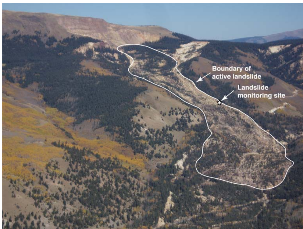
Fig. 2 Photograph showing the active part of the Slumgullion landslide and the location of monitoring equipment. Average width of the landslide is about 300 m and total length is 3.9 km
