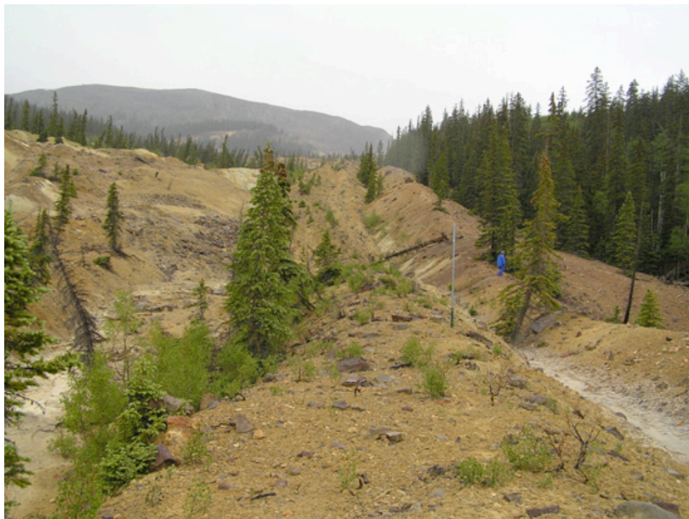
Figure 5. Flank ridges along the southern margin of the Slumgullion landslide (landslide is left of the ridges). Photograph by Giulia Biavati, Università di Bologna, Italy.
