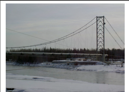
The Alaska Pipeline, here crossing the Tanana River, would offer good training for Air Force pipeline protection missions.
