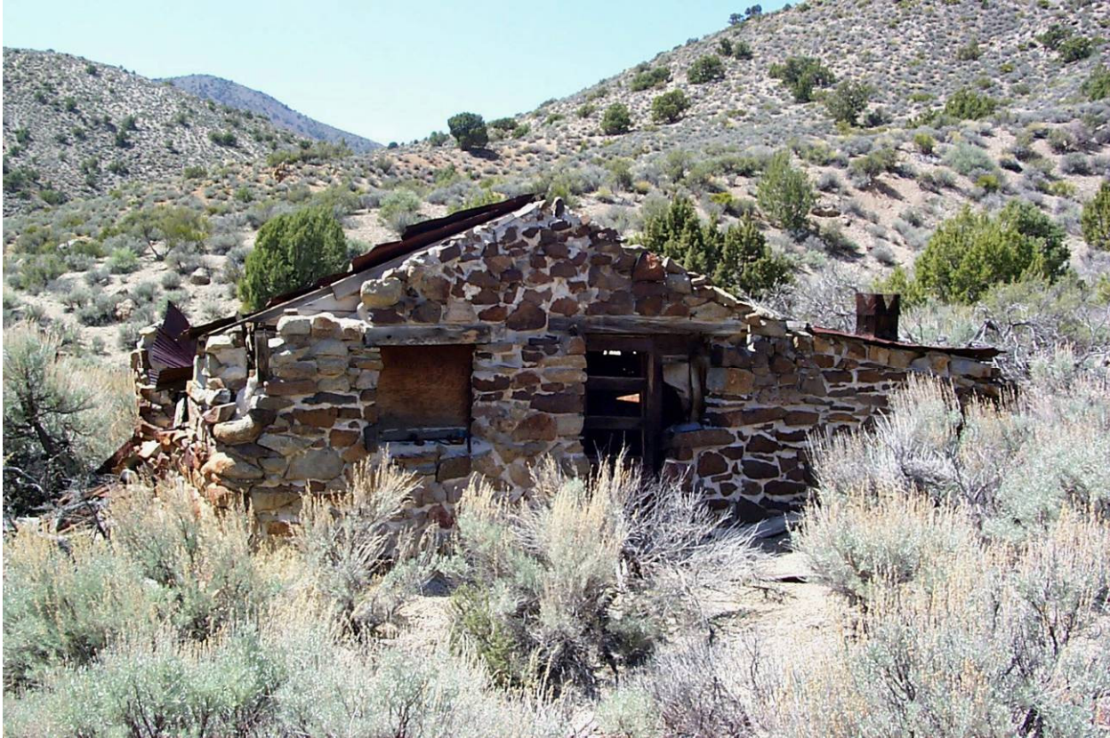
Figure A-24. Bower cabin on the NTS (photo taken by DRI, 2001)
