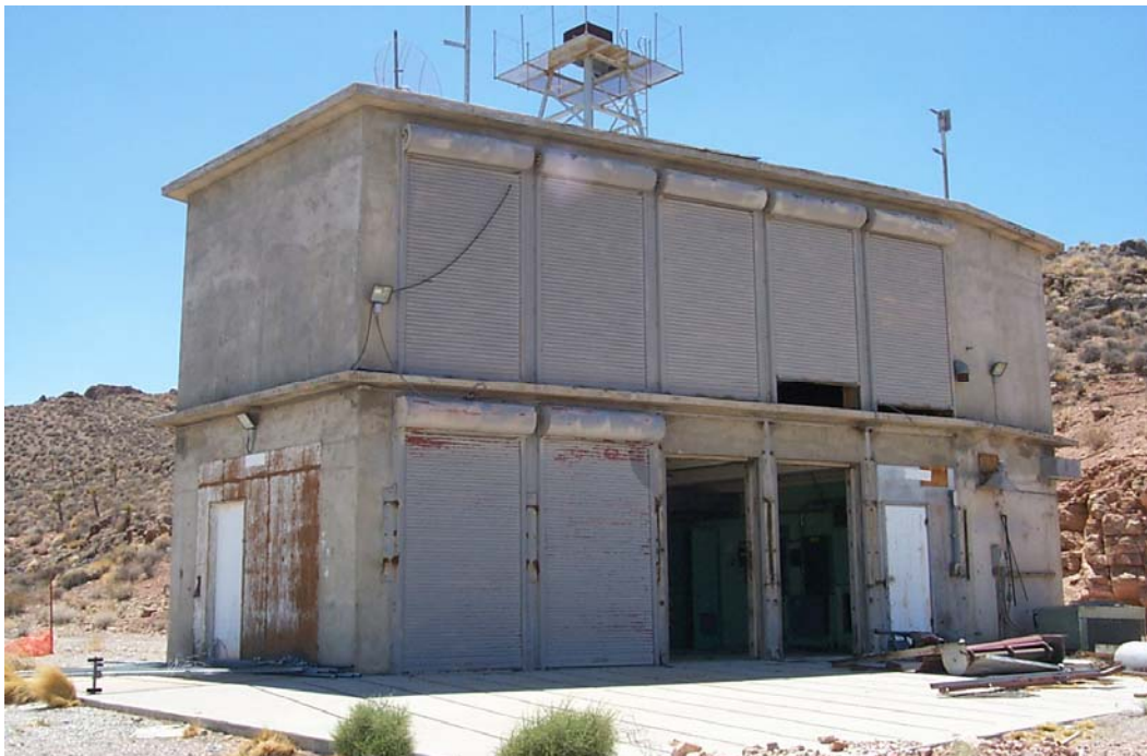
Figure A-19. Building 400, a camera station for photographing atmospheric tests, at Area 6 Control Point, built in 1951. One of the first buildings constructed on the NTS to support weapons testing activities (photo by DRI, 2003).
