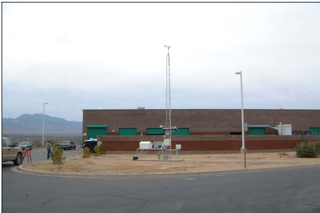
Figure 7-2. CEMP Station at Mesquite, Nevada
