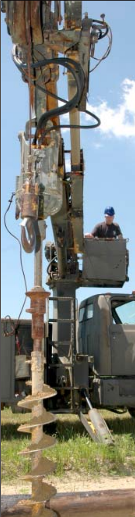
Left, Master Sgt. James Nichols, NCOIC of the electrical section, bores a hole to set a telephone pole for use in training CE members. Above, Staff Sgt. Howard Campbell, an electrical systems craftsman, hooks a piece of cable cinched around a telephone pole to a hook so the pole can be raised into position and set.
