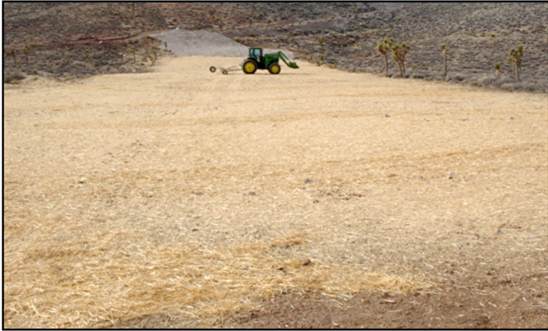
Figure 8-3. Crimping straw mulch at the CP waterline revegetation site (Photograph by D.C. Anderson, December 7, 2009)
