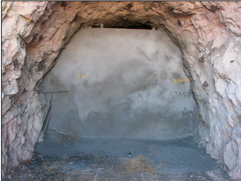
Figure 6-8. Bat-compatible closure at 16A Tunnel (Photo by D. B. Hall, December 10, 2008)
